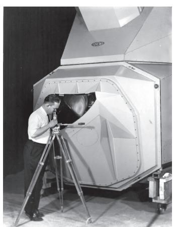
Seen at left is one of the Infinity Display Projectors that fit over the LEM simulator. A separate unit was required for each window of the spacecraft. You can imagine why the astronauts affectionately dubbed the full collection of simulators for the Apollo mission "The Great Train Wreck!"
